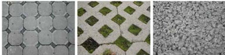
Permeable Interlocking Concrete Pavers (PICP)    Concrete Grid Pavers (CGP) "Turfstone"    Porous Concrete (PC)
