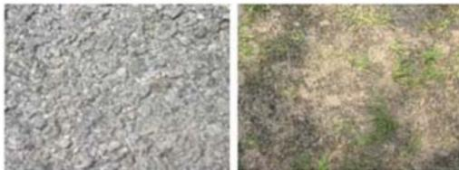
Porous Asphalt (PA)    Plastic Turf Reinforcing Grids (PTRG)
